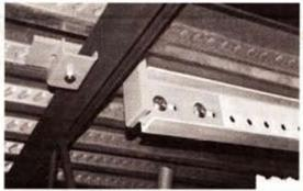
The Framing Clamp System was developed to be easily installed with the roof decking in place.
